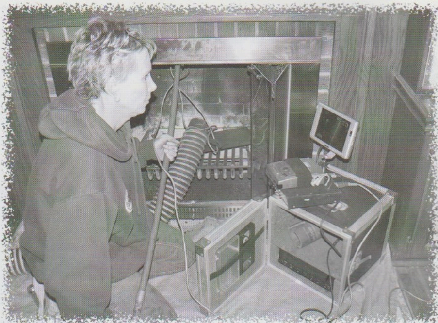
Janie scanning the flue with a Chim-Scan.
